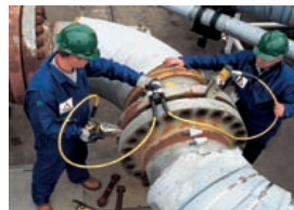
Two ENEFSH14 spreaders used simultaneously with Enerpac handpump & hoses.
