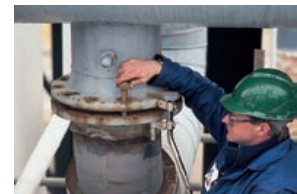
Flange alignment with ENEATM1
